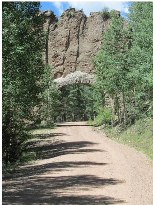
Figure 1.7. Dike with archway cut through it for road. Location is southwest of West Spanish Peak. View is westward.
